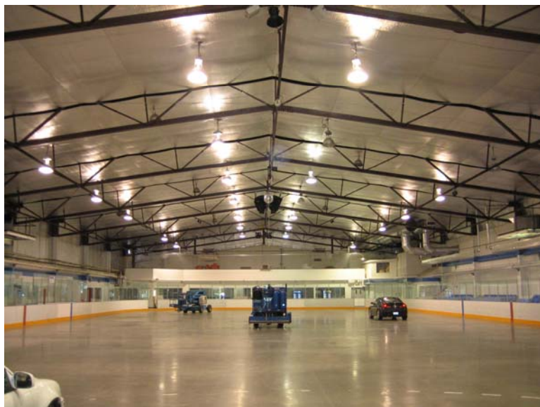
Tsawwassen BC Arena Before & After Installation Of The Low Emissivity Ceiling
